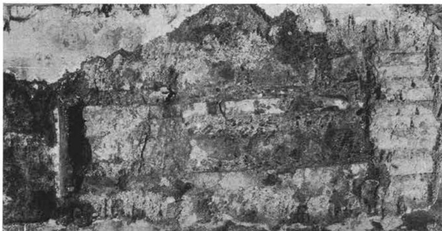
Fig. 156 — S. Lorenzo in Lucina. North wall of room to west of chancel. Right, fragment of brick wall. Center, opus listatum (Photo: Sansaini).
